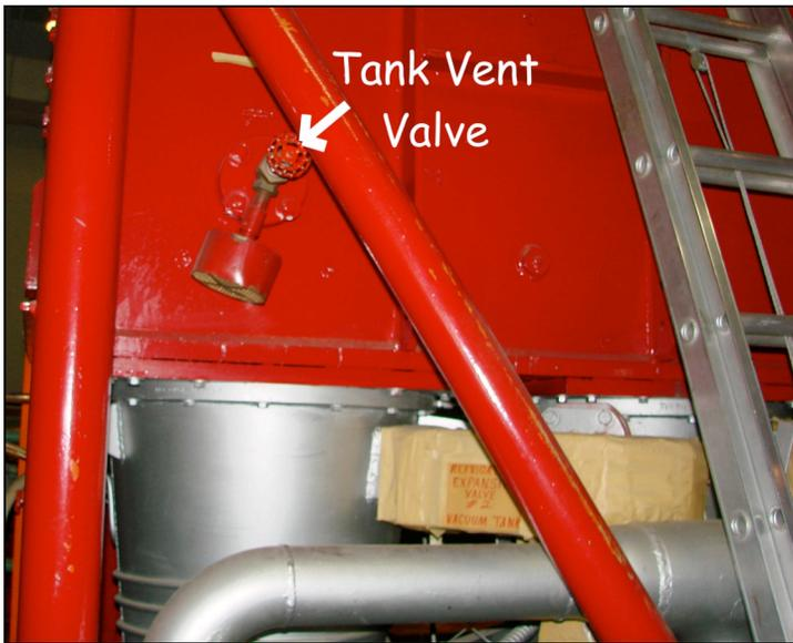
While warming the DP's up you can open the tank by first venting the tank opening the "Tank Vent Valve" then remove the two tank flange bolts that are holding the tank closed.
